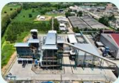
Biomass Cogeneration 120,000 mWh
